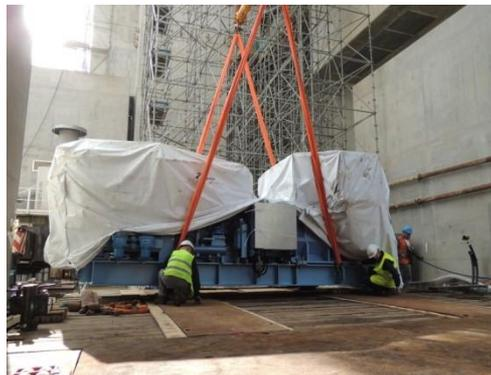
Entry of the last diesel engine for the SBO diesel generator in the northern diesel building
