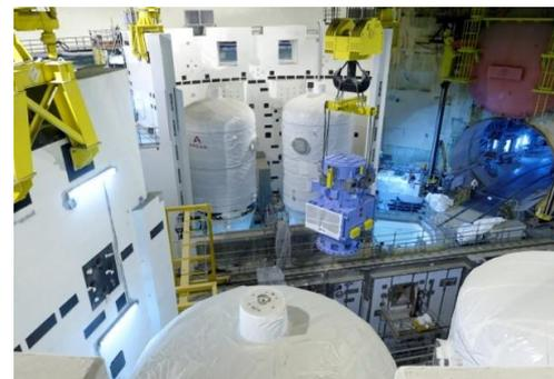
Entry of the motor for the first of the 4 reactor coolant pumps
