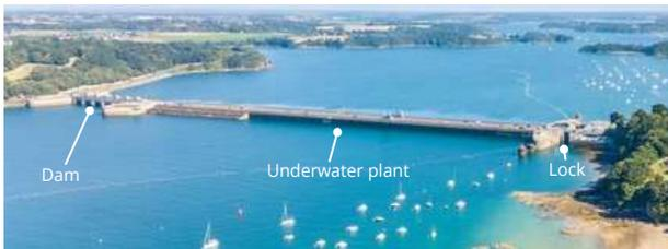
**Plant:** 390m long | 33m wide | 24 electricity generator sets of 10 MW each.
