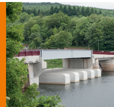
La Ravière Dam, view from upstream, creation of a flood discharge system in the form of Piano Key Weir (PKWeir).
