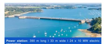
**Tidal barrage:** 115 m long l 6 valves: 10 m high - 15 m wide. **Lock:** 65 m long l 13 m wide l 15,000 vessels every year.
