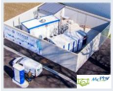
In Sarreguemines, an  $H_2$  refuelling station including an on-site AEL electrolyser was implemented in 2017 by McPhy, and operated by the city. EDF R&D analysed the performance of the installation by creating a remote monitoring and control system. The refuelling station (120 kW) delivers 350 bars for about a dozen vehicles.
