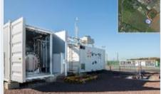
To support the development of on-field H<sub>2</sub> production and uses, this platform allows testing and qualifying electrolyzers at the megawatt scale (up to 10MW). Various of electricity sources (renewables, grid mix) can be used. H2 compression and storage is under development. Ultimately, R&D in e-fuels will be carried out.
