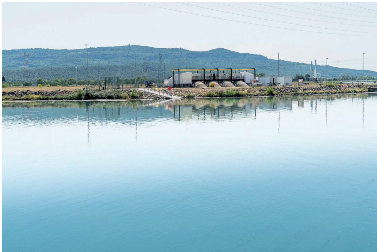
Station de pompage
