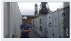
In 2020, EDF R&D provided its expertise for the verification of acceptance tests of 5MW/30min stationary battery in Guadeloupe. The operational battery responded successfully to the frequency control service designed by EDF R&D.
