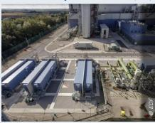
49MW battery storage facility at the West Burton power station site was the largest project in the regulation system that had been set up across the UK. This system improves the stability of the electricity network enables a rapid response to frequency fluctuations.
