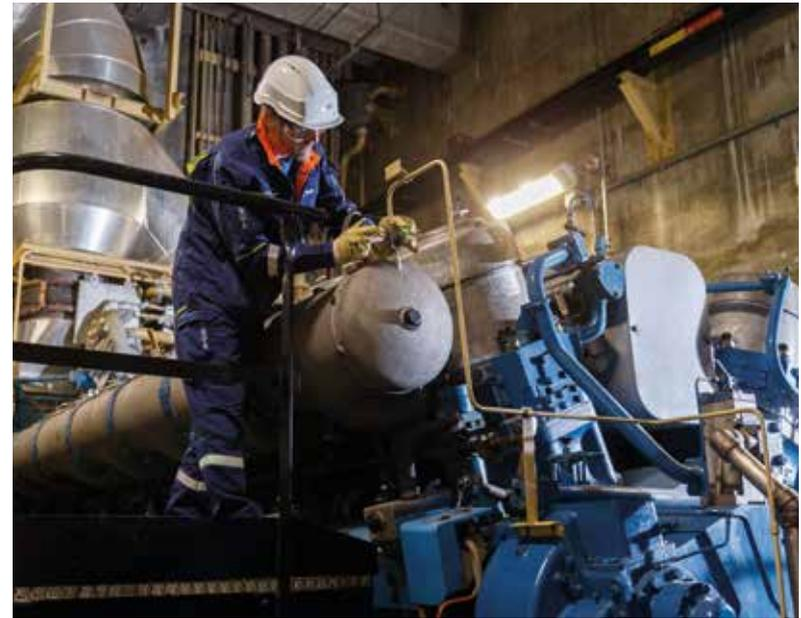
*Maintenance on a emergency diesel generator*
