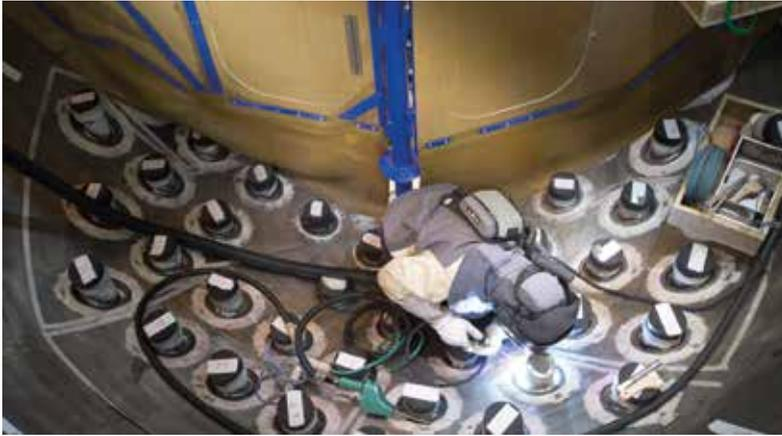
Welding of vessel head sleeves
