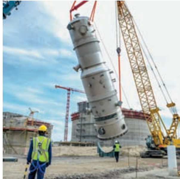
Lifting a condenser on the LNG terminal construction site, Dunkirk, France.
