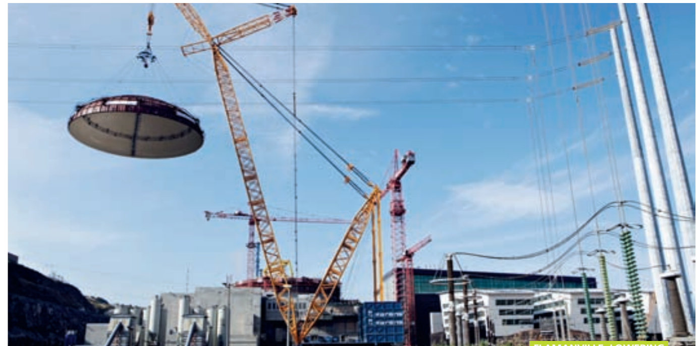
FLAMANVILLE: LOWERING THE 260 TONNE DOME ONTO THE EPR
