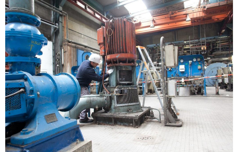
Pump maintenance in a thermal power plant
