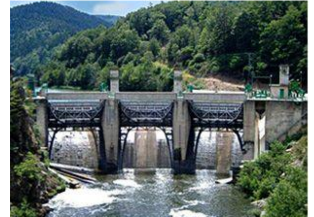
The Poutès dam currently.
