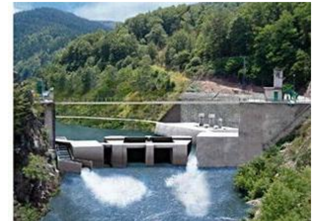
The dam following redevelopment.
