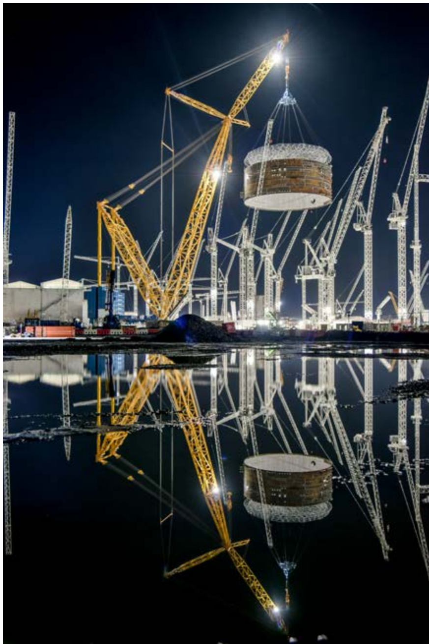
Unit 1 containment ring lift - Hinkley Point C construction site
