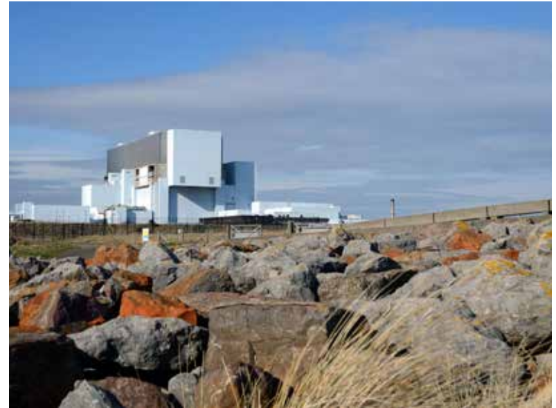
Torness nuclear power plant
