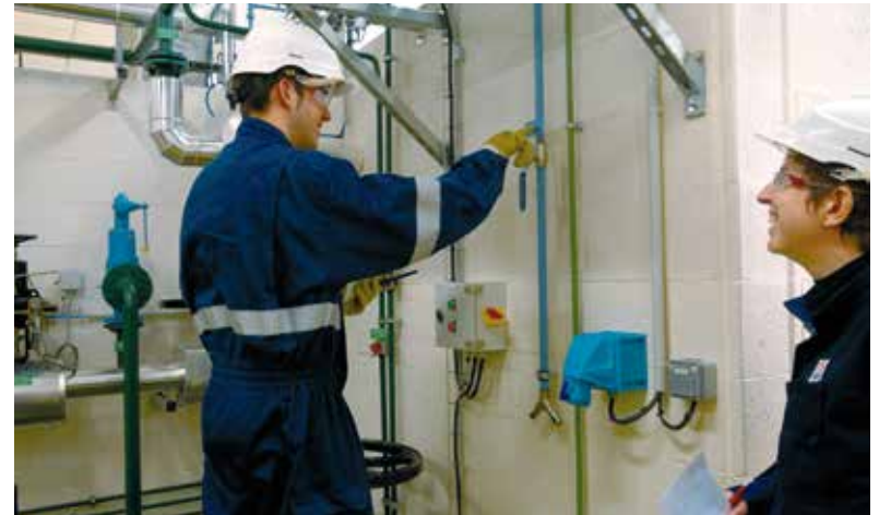
Using human performance tools - Civaux nuclear power plant
