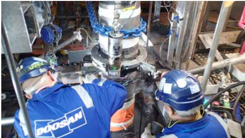
Maintenance work in an AGR
