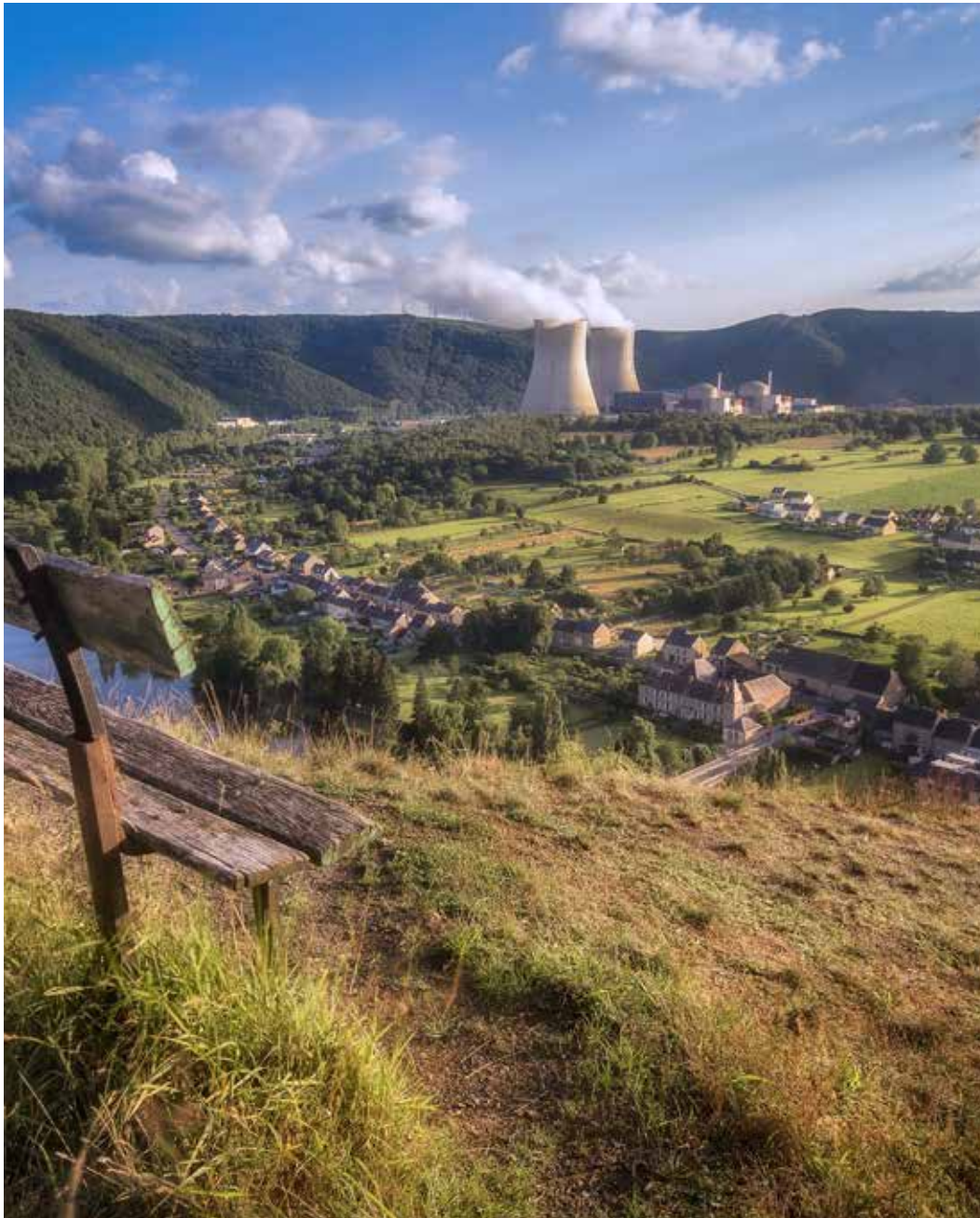
Chooz nuclear power plant
