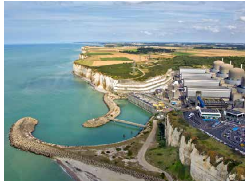
Paluel nuclear power plant
