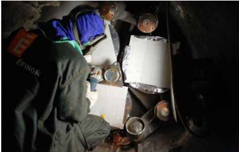
Grinding operation - Flamanville nuclear power plant
