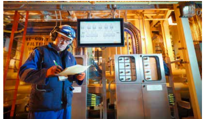
Recording parameters - Hartlepool nuclear power plant
