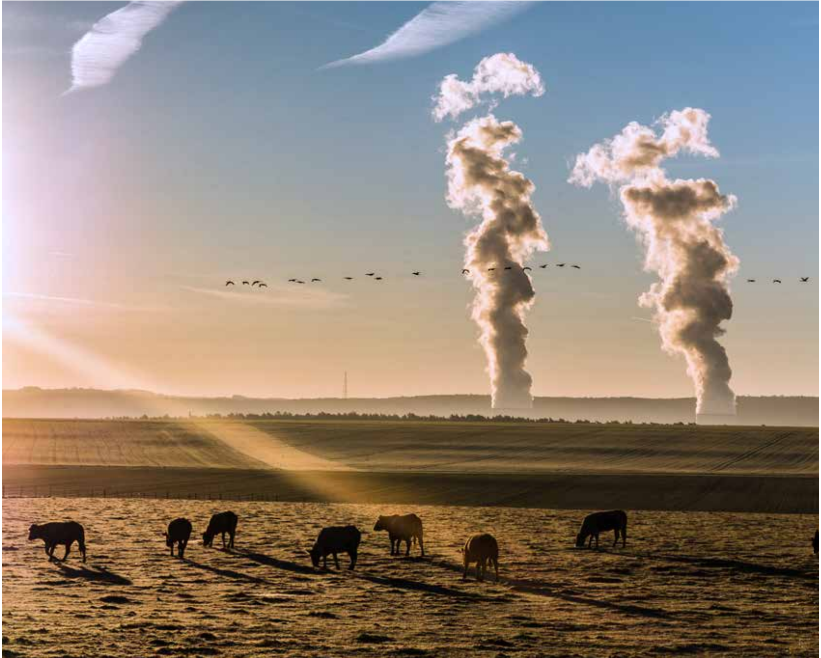
Chooz nuclear power plant
