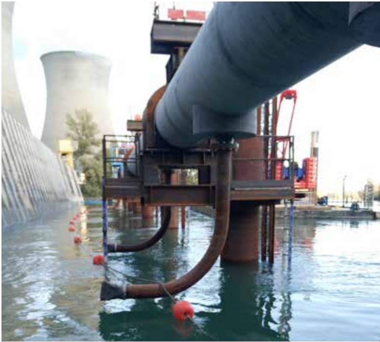
Systems designed to prevent frazil ice formation
