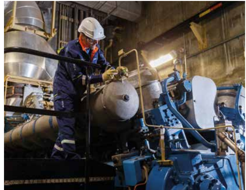
Maintenance on a emergency diesel generator
