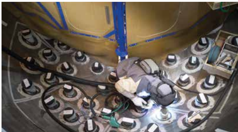
Welding of vessel head sleeves
