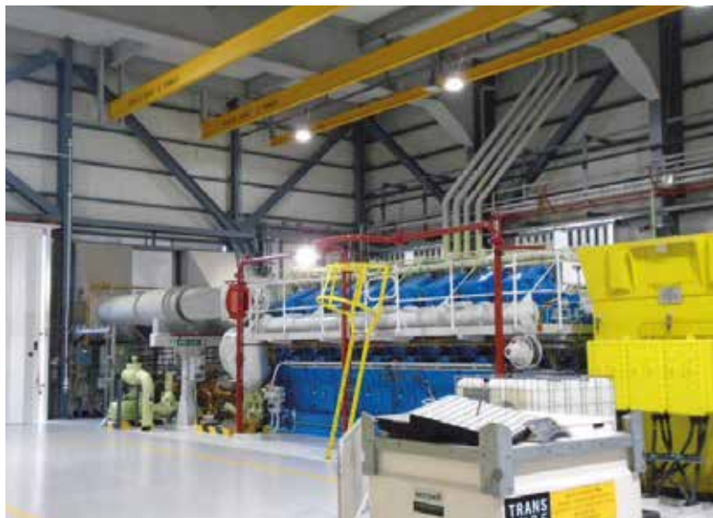
Emergency diesel generator in an AGR
