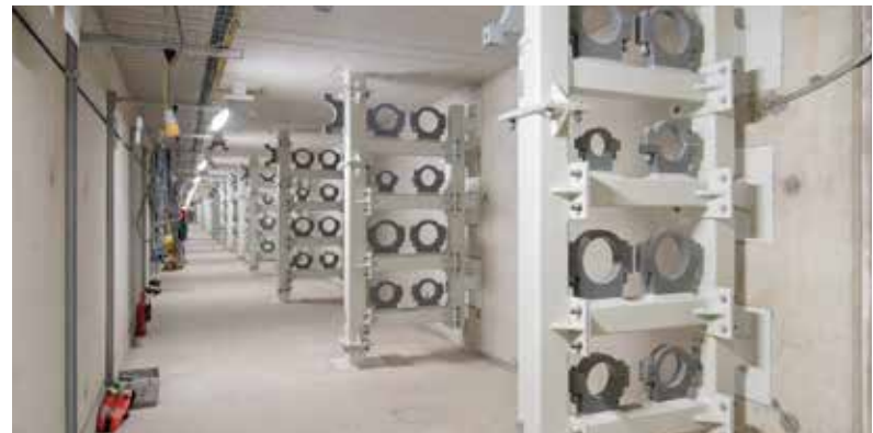
Pipe supports in a gallery - Hinkley Point C
