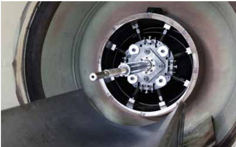
Robotic weld repair of a main secondary system pipe - Flamanville 3
