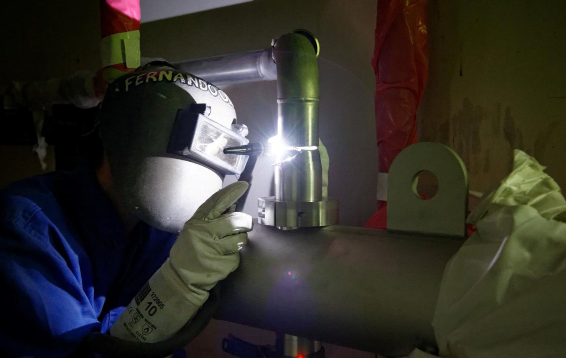
Auxiliary nuclear building Welding of an effluent treatment pipe.
