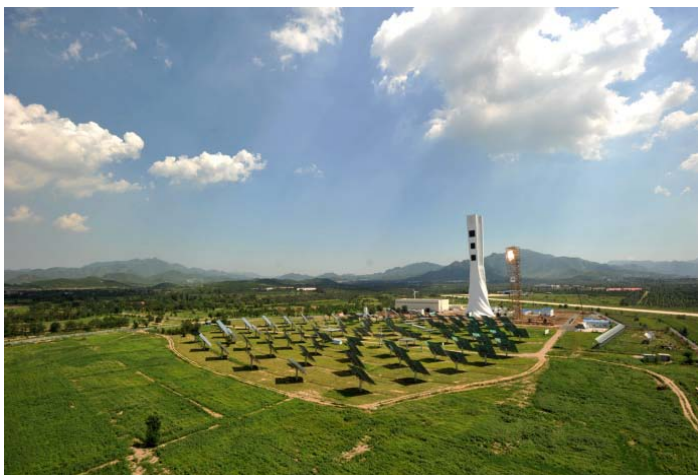
The solar concentrator tower at Badaling, surrounded by 100 reflecting mirrors.
