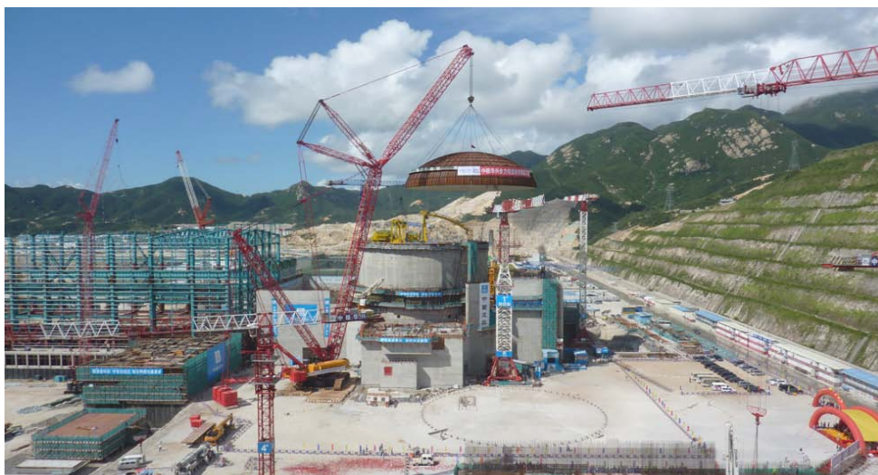
Installation of the reactor building dome on unit 2, 12 September 2012
