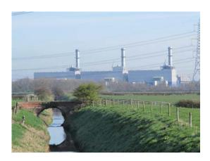
From an environmental viewpoint, the CGGTs are the best performing of all the thermal resources. Because they use gas (a fuel that is cleaner than coal or oil) and due to their exceptional output efficiency (57% against 35% for a conventional phase), they discharge less than half the CO2 of the conventional resources.
