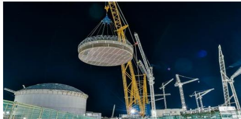
Unit 2 liner cup lifting in September 2020, 4 months faster than Unit 1
