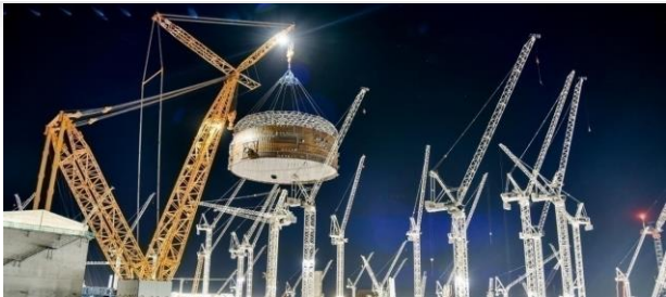
The 400 tonne liner was successfully lifted into position in Unit 1 reactor building in December
