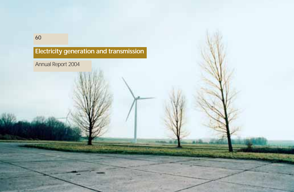
Put on stream in 2004, the Clef des Champs windfarm in the Aisne region consists of four 2.75 MW turbines, the most powerful aerogenerators to date in France.
