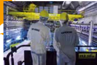
Dismantling at Chooz A.
