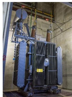
Transformer in the 63kV pumping station substation
