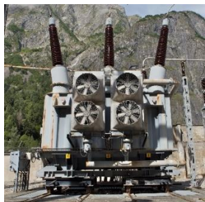
Plant output transformer
